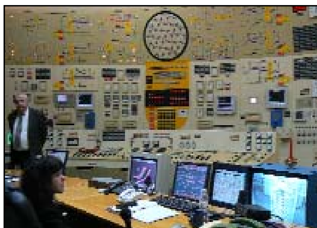
Control room of Unit 3, December 31, 2007, during shut down operations
