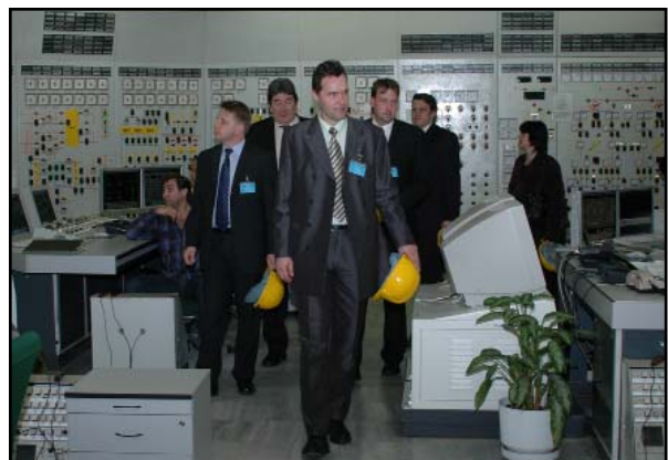
Mr Martin Klepetko in a reactor control room
